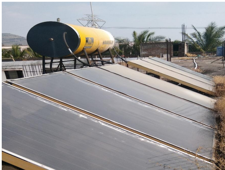
Photograph of Roof Top Solar PV Plant & Solar Thermal Water Heating System:
